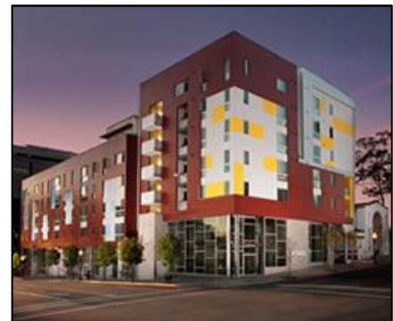
Cedar Gateway is an award-winning 65-unit affordable housing community in San Diego with 23 dedicated units for BHS clients who were formerly homeless.
